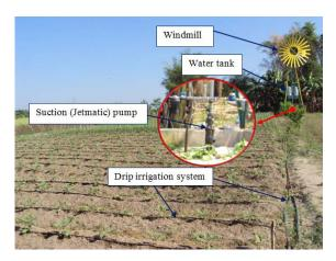
Figure 1 Windpump-drip irrigation system
